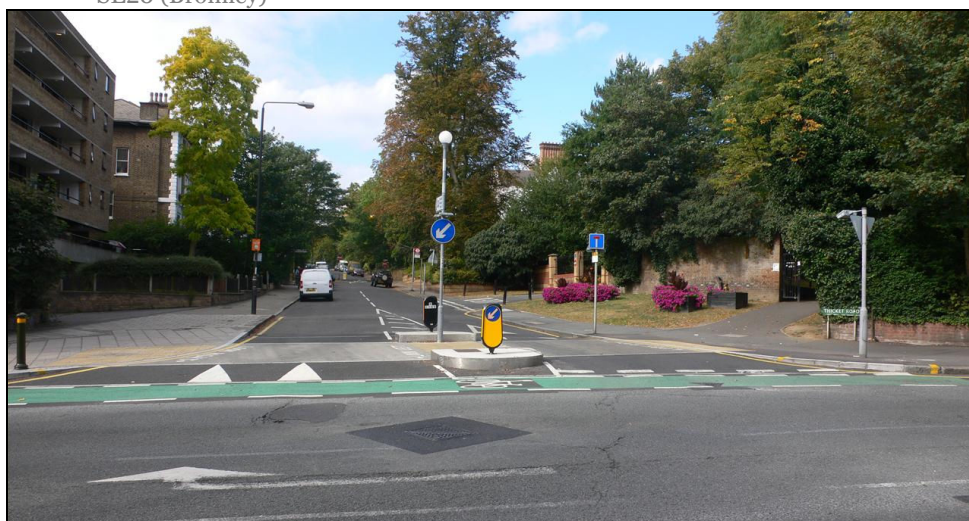
Fig 4. Entry treatment on Thicket Road at intersection with Crystal Palace Park Road, SE20 (Bromley)
