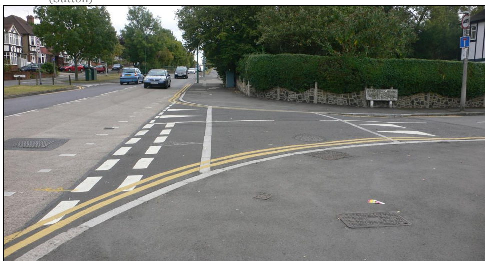
Fig 2. Entry treatment on Cranleigh Gardens at intersection with Angel Hill, SM1 (Sutton)
