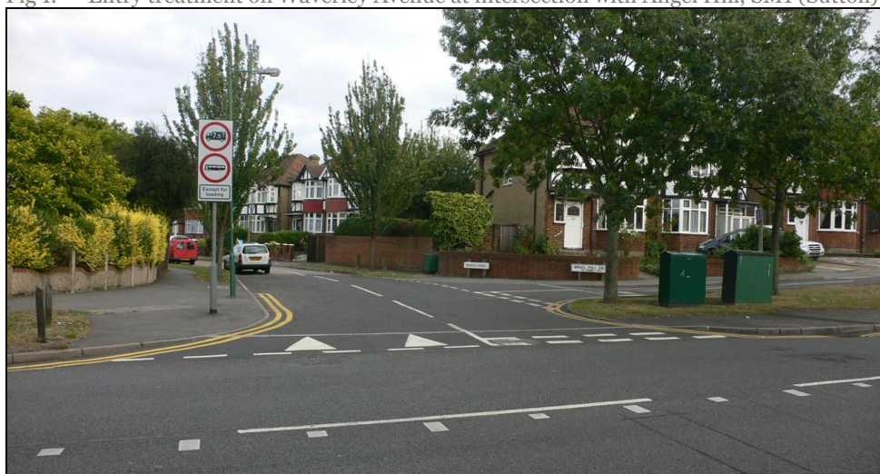
Fig 1. Entry treatment on Waverley Avenue at intersection with Angel Hill, SM1 (Sutton)
