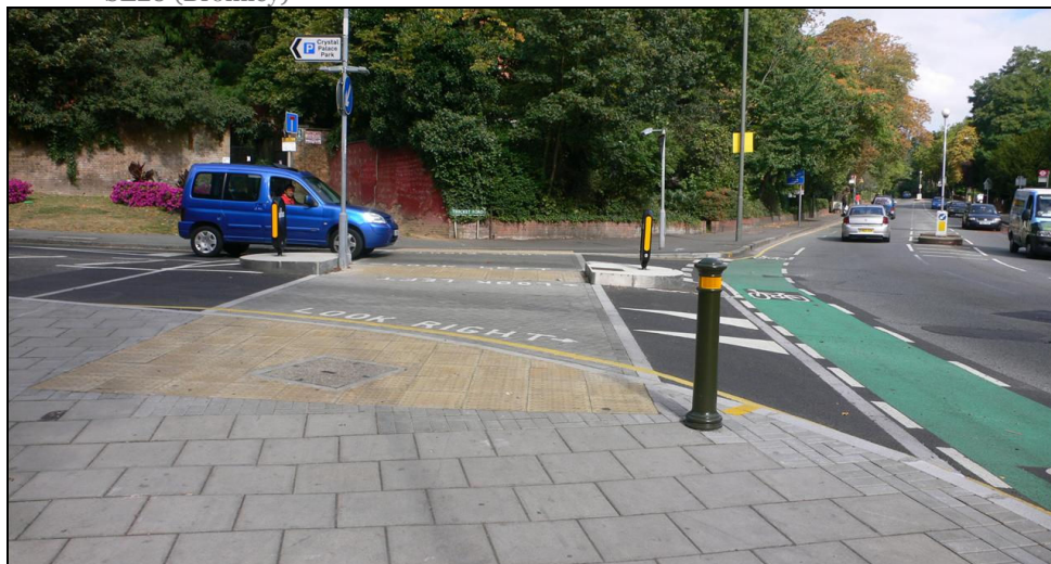
Fig 3. Entry treatment on Thicket Road at intersection with Crystal Palace Park Road, SE20 (Bromley)
